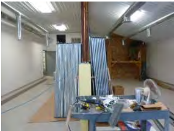
Above: Large dog kennel room. Equipment purchased through $10,000 anonymous grant, $5000 donation from Allegan Women Who Care and May 2:1 anonymous donor matching funds which raised $31,500. Installation soon.
